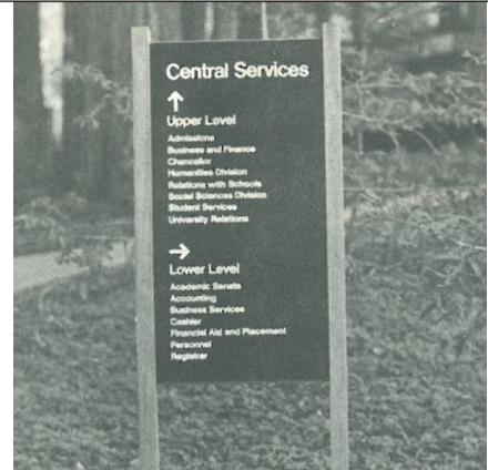
**Original:** The signs are fabricated from plastic laminate and are wall-mounted or supported by redwood posts. The type is silk-screened directly onto the plastic laminate surface and can be removed with the use of paint thinner for alterations.
