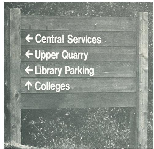
**Current:** Alupalite planks with anodized aluminum H channel with rough-cut 6x6 redwood posts; 4" Univers 67 Condensed Bold type.
